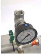
Pipe work fitting into which the pressure vessel is screwed into.
