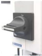
Release the screw in the side of the isolator switch knob, and remove knob.
