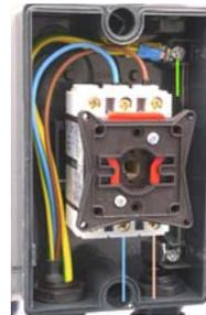
Knock out a cable entry, and fit an appropriate cable gland. Connect the single phase supply wires into isolator switch terminals as shown.
